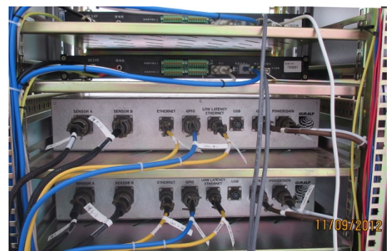
Figure 4 Digitiser setup with dual back-up CD24R6EAM
