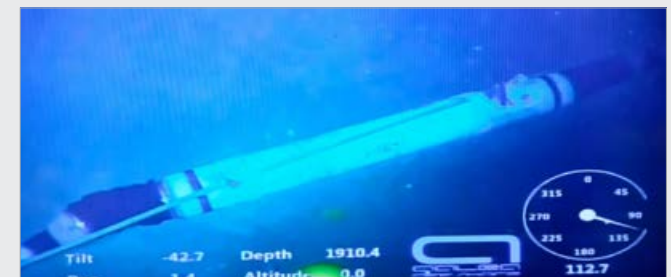
Image 20: Deployed SMART cable repeater on the seabed
